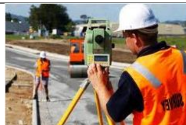
Levelling for vertical control
